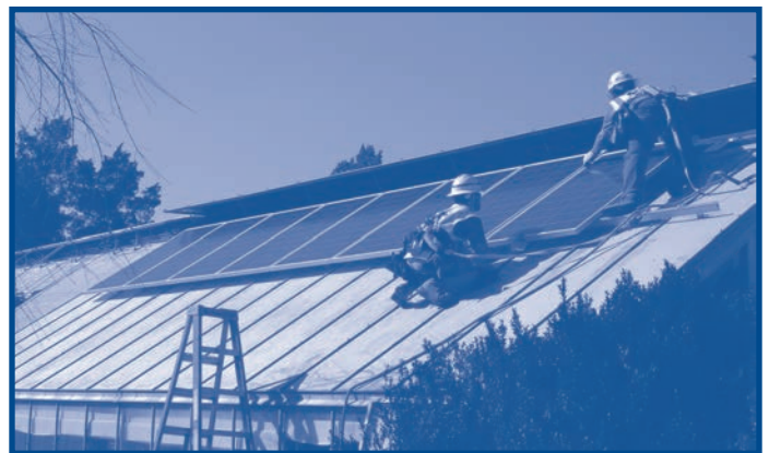
INSTALLATION OF SOLAR PANELS
